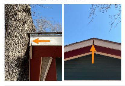
8: Improperly Installed Drip Edge
