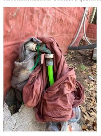
2: Sink P Trap Incorrect Installation
