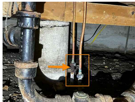
Crawlspace- Copper Pipe
