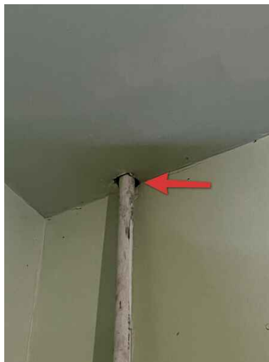
Ceiling Fire Separation
