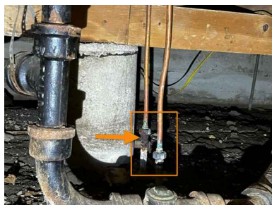
Crawlspace- Copper Pipe
