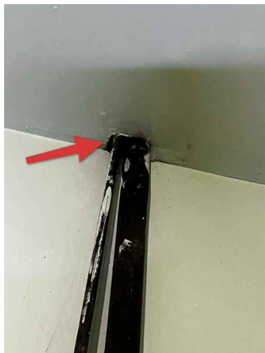
Ceiling Fire Separation
