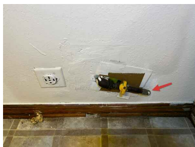
Kitchen- Gas Pipe
